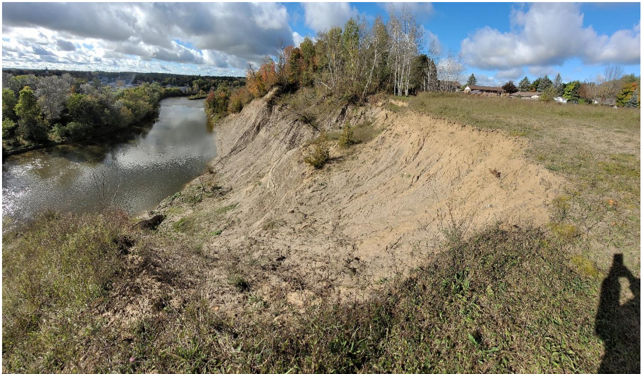
Erosion at the top of the bank ▼
