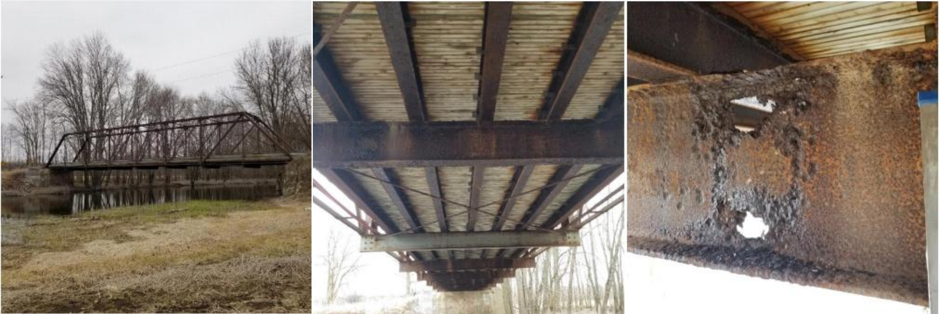
Figure 97 Example of Bridge in Very Poor Condition
